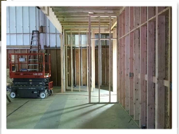
Framing the walls inside the new community room
