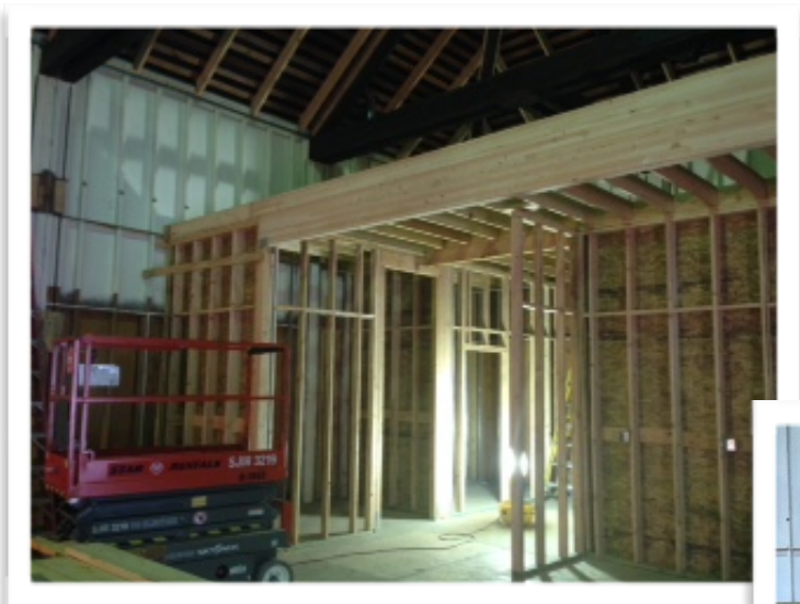
Framing the walls inside the new community room
