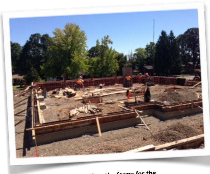
Assembling the forms for the footings for the new gym
