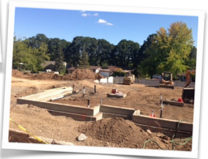
Foundation footings for the new gym
