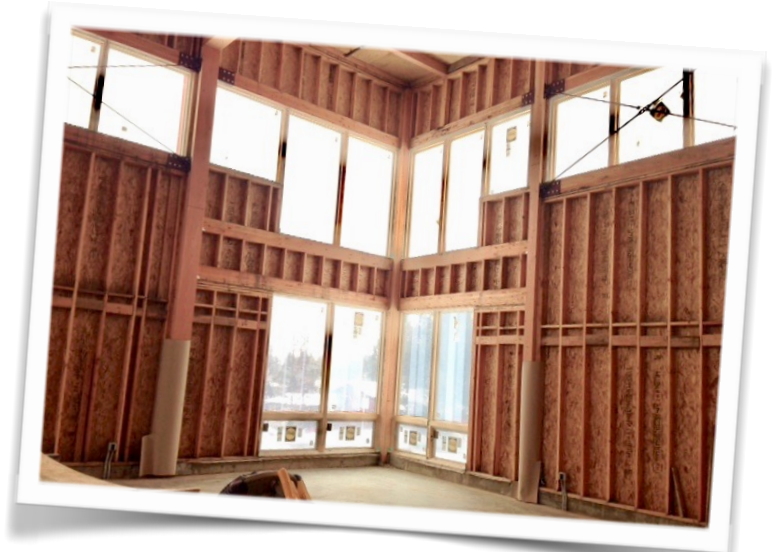
Interior southwest corner of gym with windows installed.
